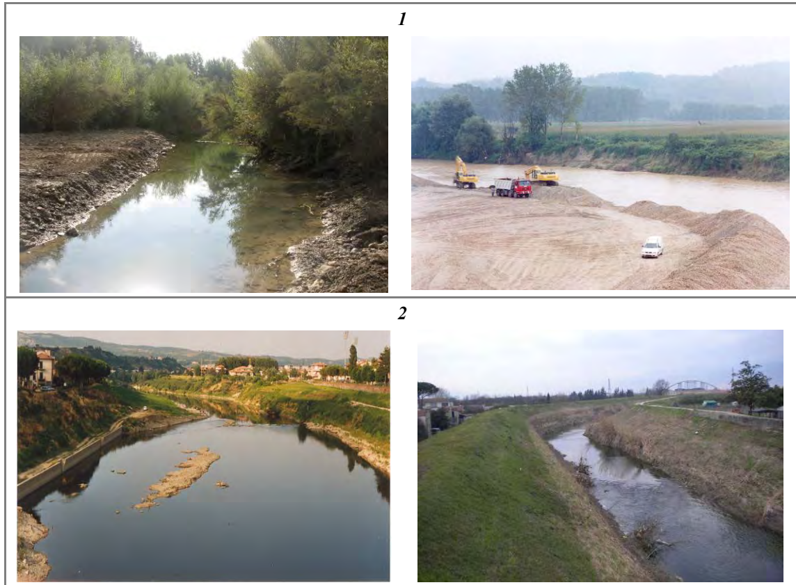
Figure 40 – Alteration of cross-section variability in partly- and unconfined channels. (1) Cases of partial homogenization of the cross-section due to interventions. (2) Cross-section homogeneity extended for long reaches due to excessive artificiality.
