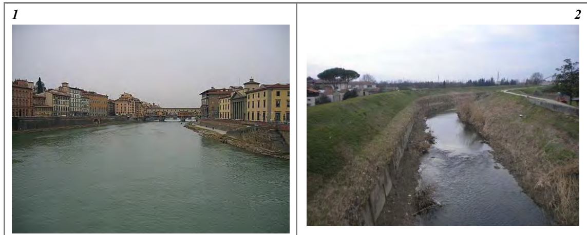
Figure 70 – Cases of bank protections plus levees in contact occurring for most of the reach (> 80%), for which a score of 12 is added.
