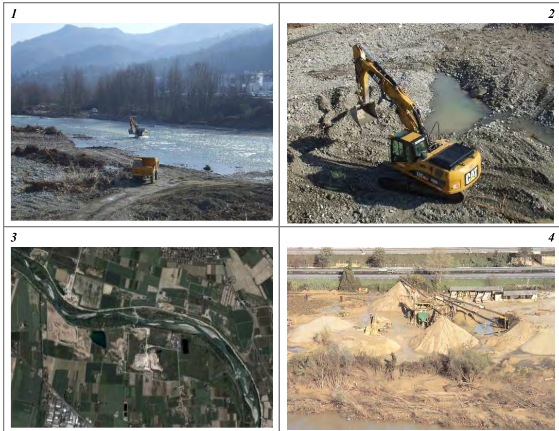
Figure 75 – Sediment removal. (1) and (2) Recent and present activity; (3) and (4) indirect indicators of intense past activity are the presence of mining sites. Assignment to Class B or C depends on the extension of the activity (localized or widespread), in the case of confined channels, and on the intensity of the mining activity either in the past and in recent times, in the case of partly- and unconfined channels.
