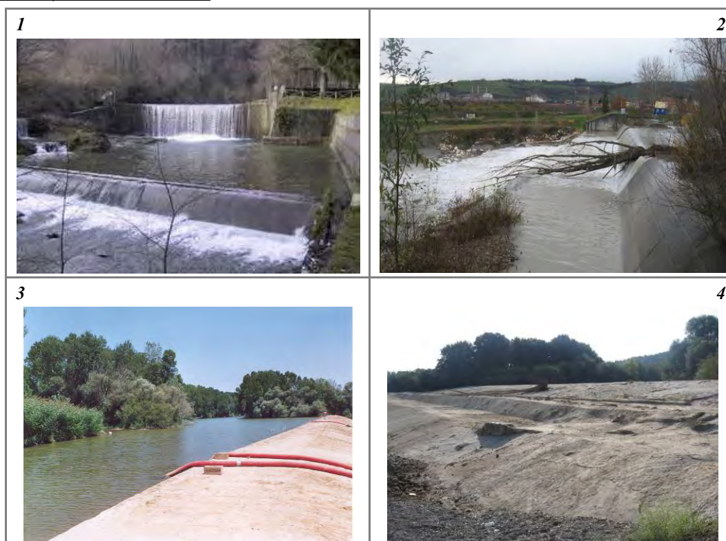
Figure 56 – Transversal structures of alteration of sediment discharges in hilly and lowland areas. (1) Consolidation check dam; (2) abstraction weir; (3) not filled abstraction weir; (4) filled abstraction weir.
