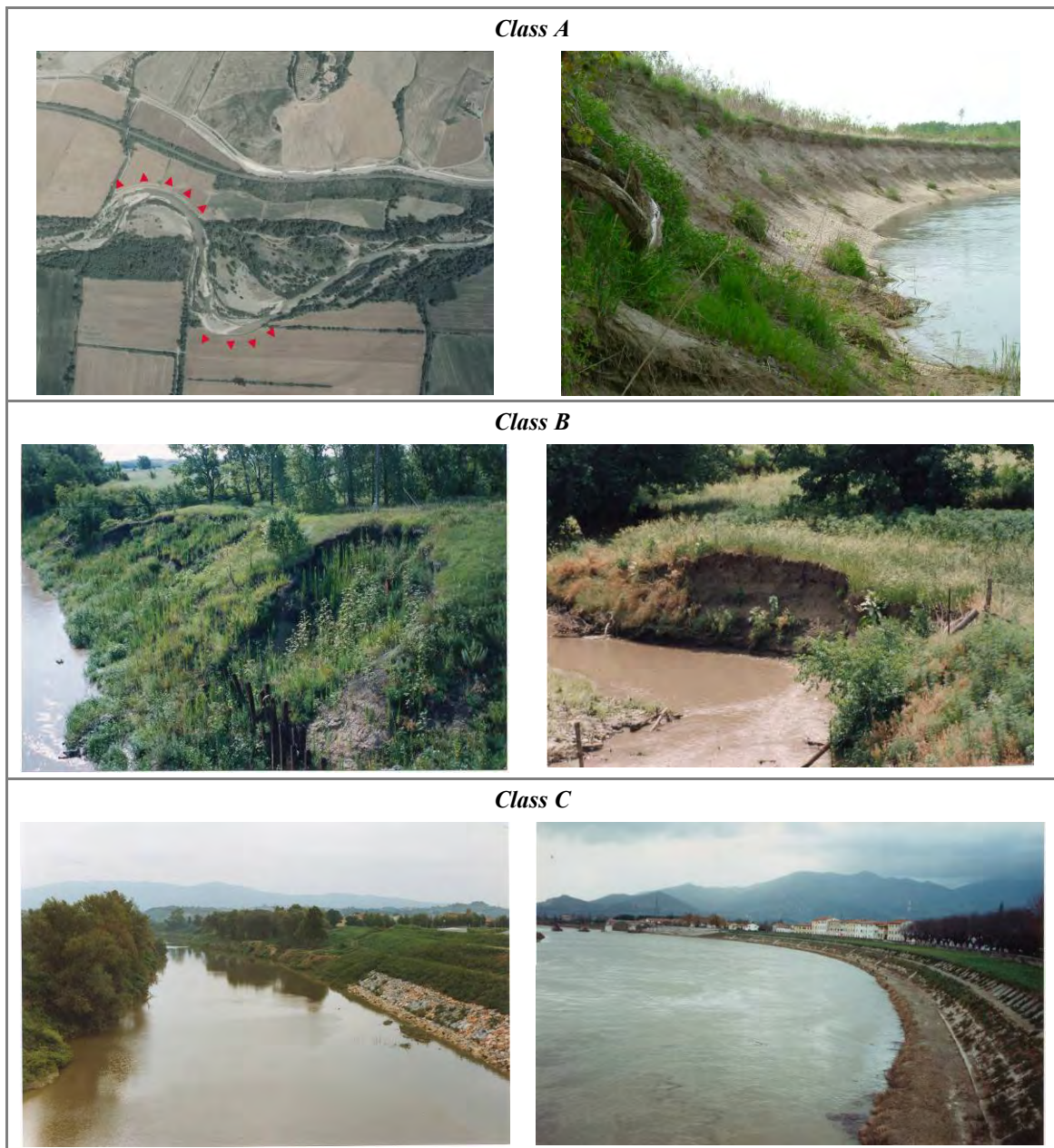
Figure 32 – Processes of bank retreat. Class A : frequent retreating banks, particularly along the outer side of bends (red arrows, photo on the left). Class B : this class includes reaches with bank erosion observed only locally. Class C : absence of eroding banks due to bank protections and/or absent channel dynamics.
