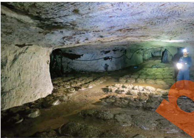
Fig. 24 - Gallerie di cava adibite a fungaie. - Quarry tunnels used for mushrooms cultivation.
